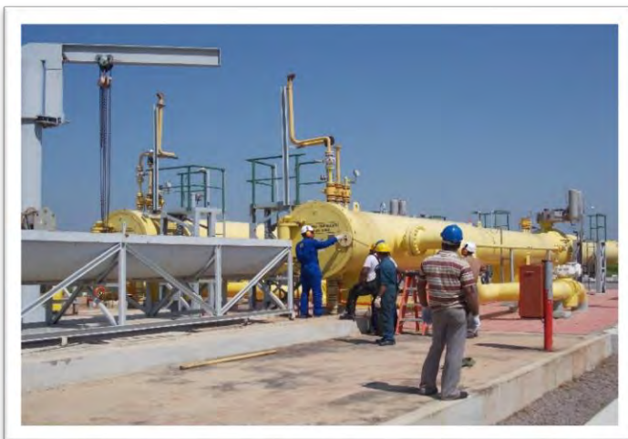
Pig Launcher and Receiver – CS5
