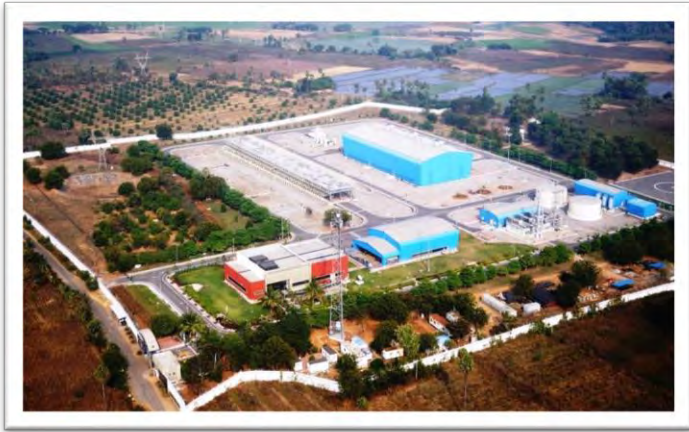
Aerial view of compressor station – CS 3
